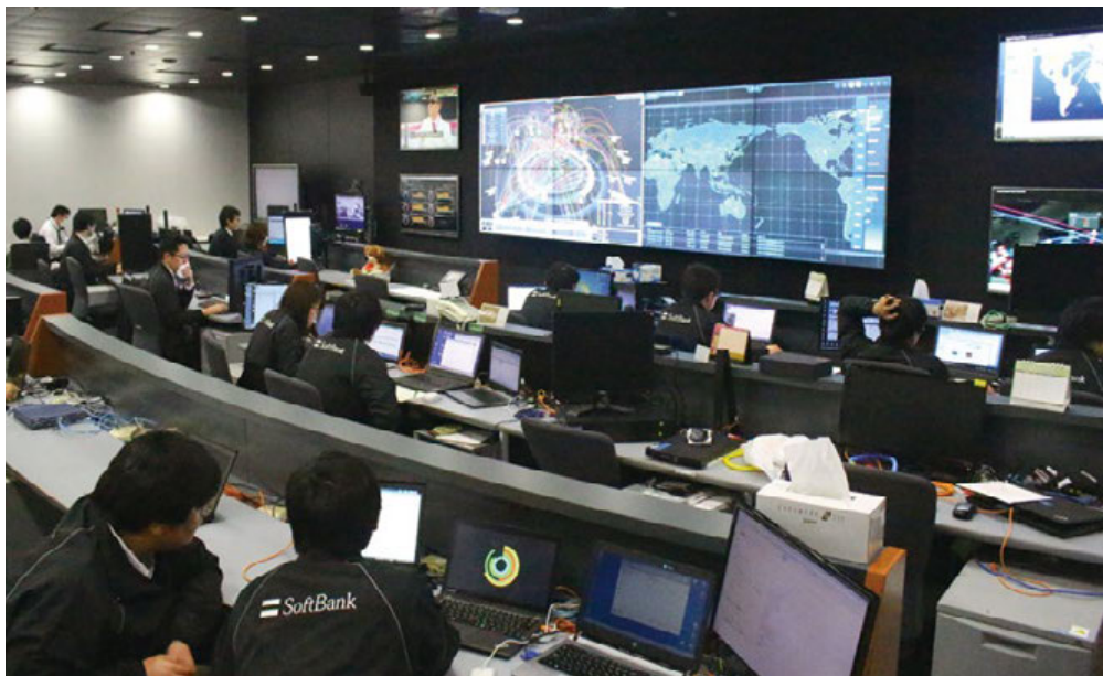
Security operation center
