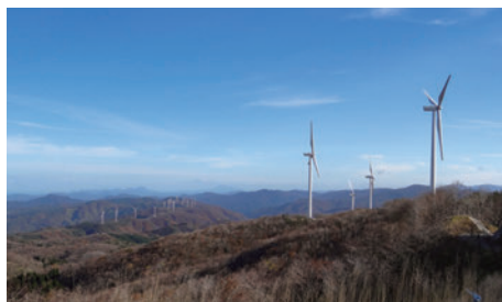
Wind Farm Hamada
