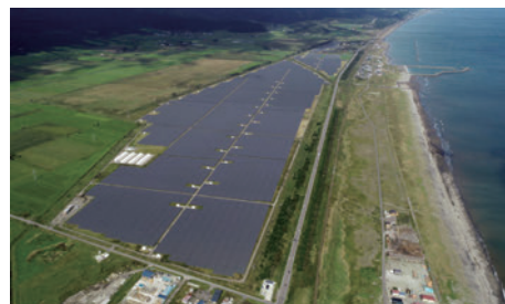
SoftBank Yakumo Solar Park
