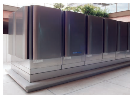
Industrial fuel cell power generation system Bloom Energy Server
