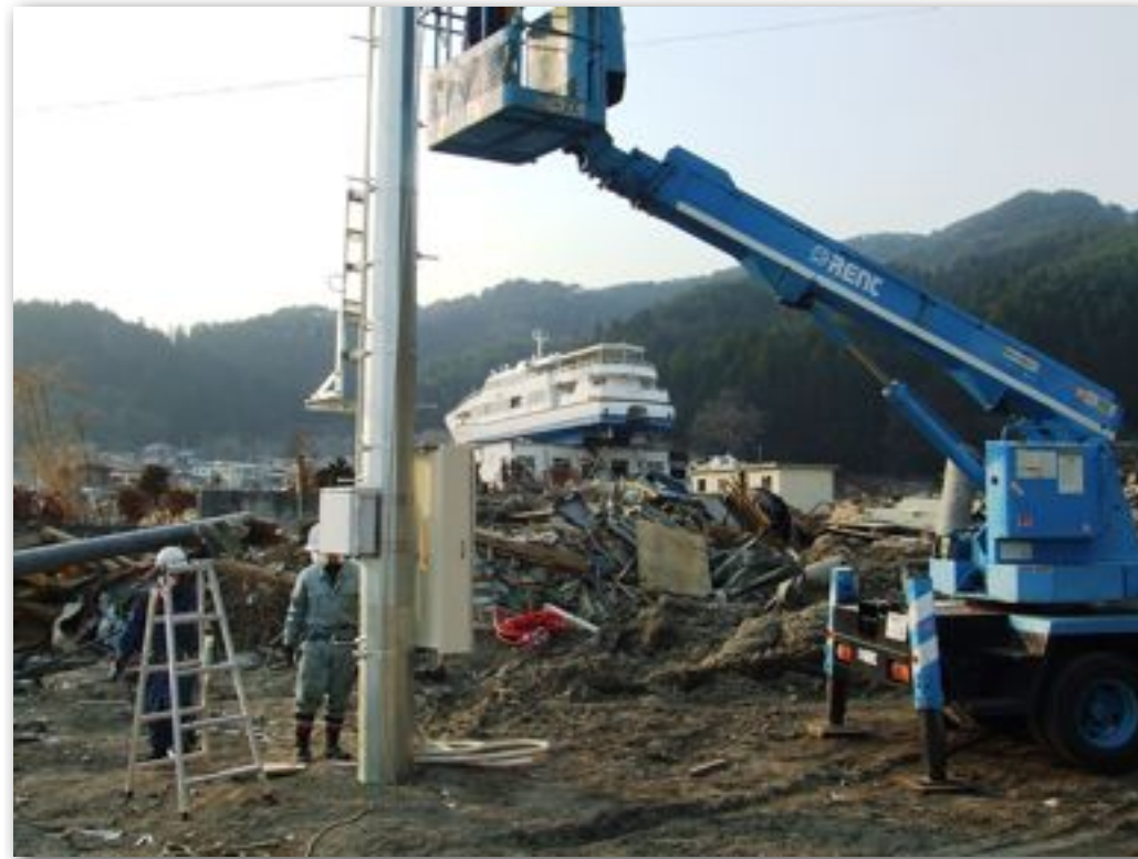
Restore base stations
