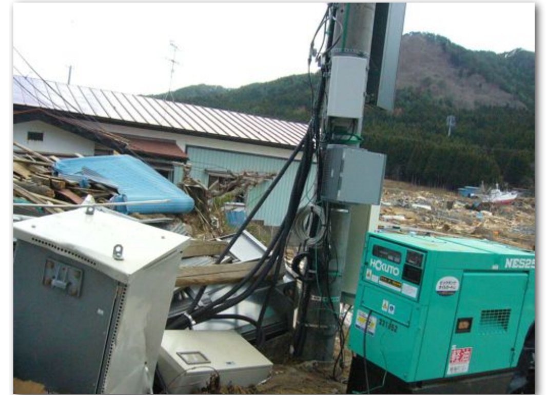
Placement of power generators
