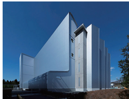
Environmentally conscious next-generation data center
