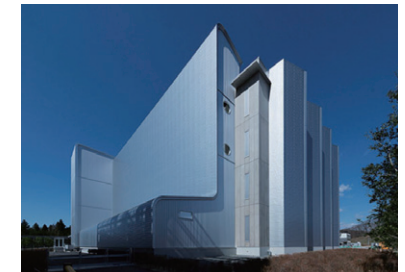
Shirakawa Data Center
