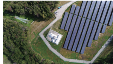
Miyagi Osato Solar Park
